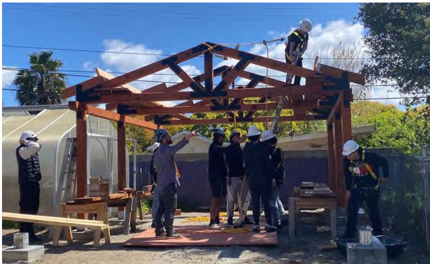
(Redwood HS Construction Pavilion project)
