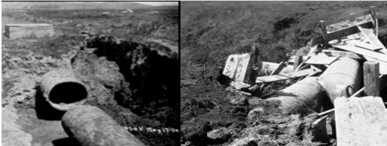
Figure 2: Water Mains Damaged by the 1906 San Francisco Earthquake
