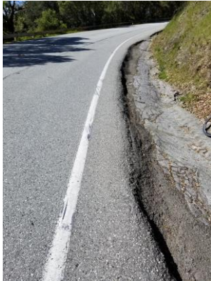
Figure 8: Narrow shoulder of Highway 35 north of Crystal Springs Road
